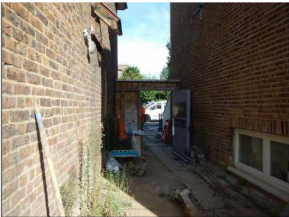
Image 3 – view of access from Shaftesbury Road
