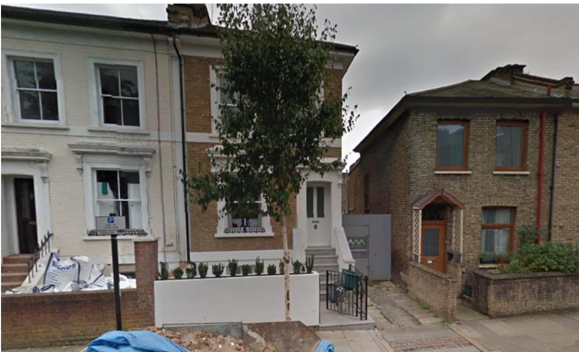
Image 1 – Frontage of No. 6 Shaftesbury Road with access to application site between No. 4 and 6 Shaftesbury Road
